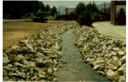
A. Riprap solves the erosion problem at the expense of the stream's natural beauty.
