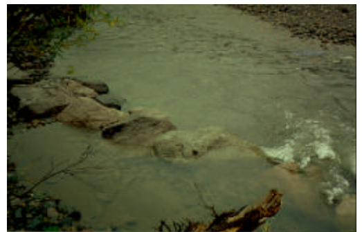
D. Rock vanes deflect the force of the stream away from the streambank.
