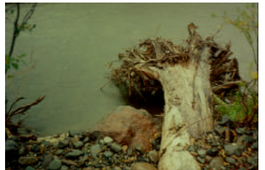
C. Rootwads armor the bank, deflect flow and create fish habitat.
